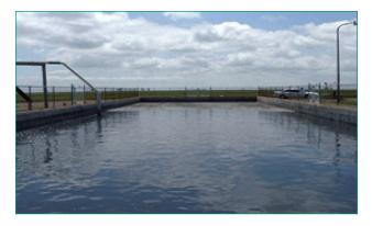
**Fig 2:** After 47 days of treatment most of the surface scum and bottom solids have been eliminated.
