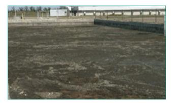
**Fig 1:** After 26 days of treatment the crust shows evidence of bubbling and chunks of sludge being brought to the surface.
