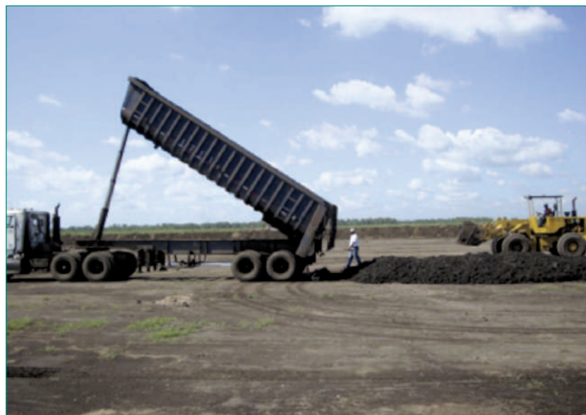
Fig. 2: This picture depicts placement of the windrows.
