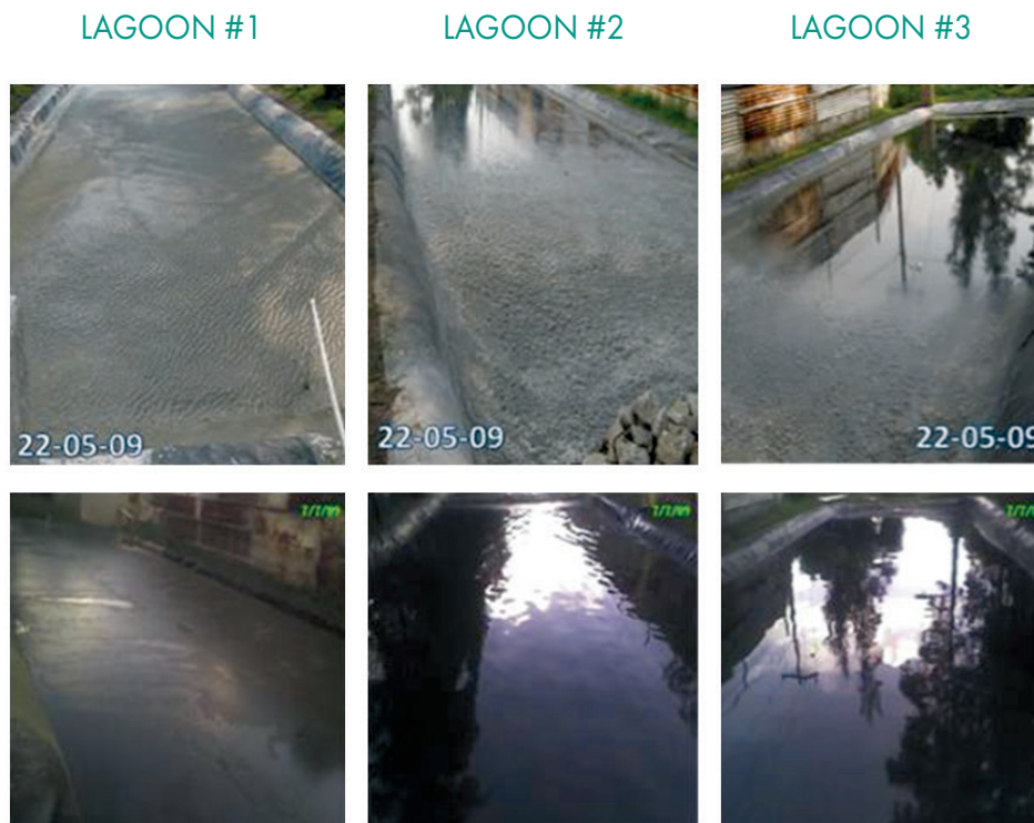
Fig. 1: These pictures taken on 5/22/09 (above) and 7/1/09 (below) show the condition of the three lagoons after treatment compared to during treatment. Note the condition of the lagoons improve from the first to the third lagoon in the series.
