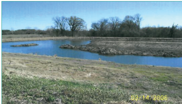
Fig. 3: This picture shows the site after successful remediation.
