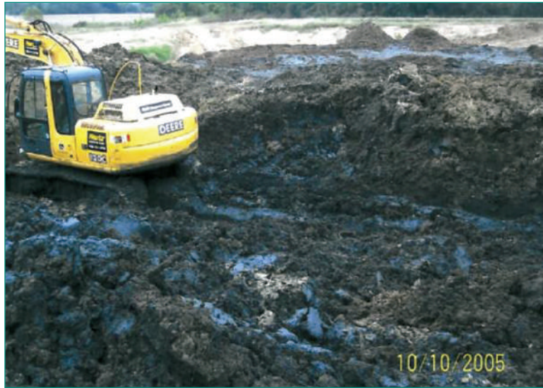
Fig 2: Excavation to ready the site for land farming shows the extent of contamination.
